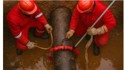
The tool's long handle provides good leverage, allowing it to snap pipes squarely before the cutter wheels penetrate halfway. It offers a clean cut and can be used in tight spaces like ditches, underwater, noise-free zones, overhead, and in pipe racks. It operates with minimal rotation (45 degrees) and is suitable for cutting steel, cast iron, galvanized, ductile iron, black iron, and stainless steel pipes.
